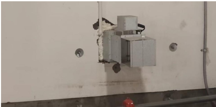
Three-way discharge structure
