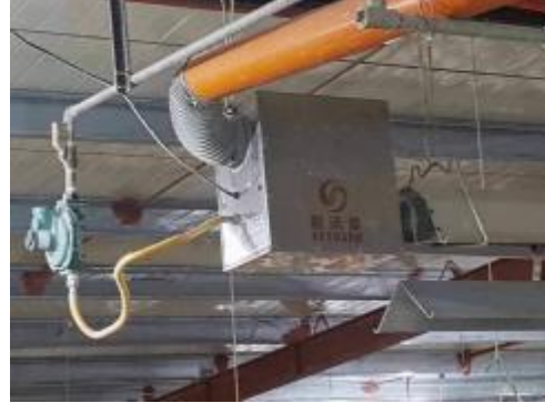
Equipment and gas-supply connection details
