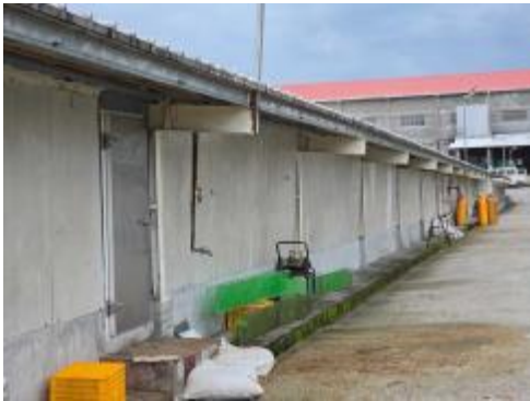
Overall exterior view of the broiler house and propane tanks
