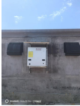
Outdoor heater installation
