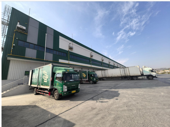
Exterior facade and doorway area
