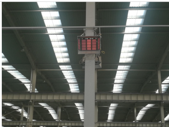
Close-up of HTC09 ceramic plaque radiant heater installation
