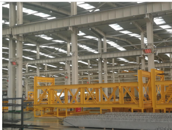
Multiple heater arrangement inside the large industrial space
