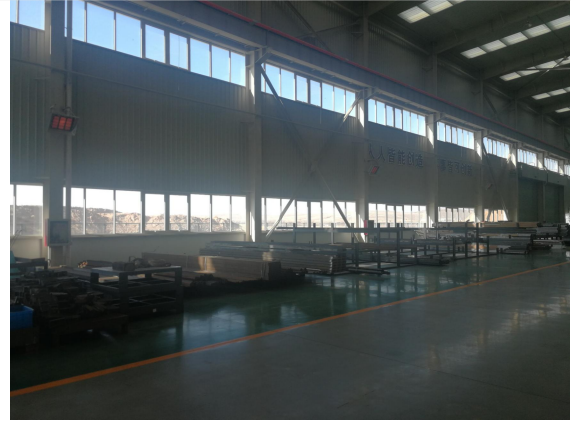
Side-wall zone and localized radiant heating scene
