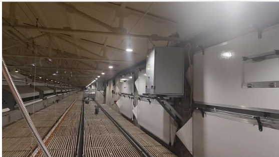
Actual installation of the units along one side wall
